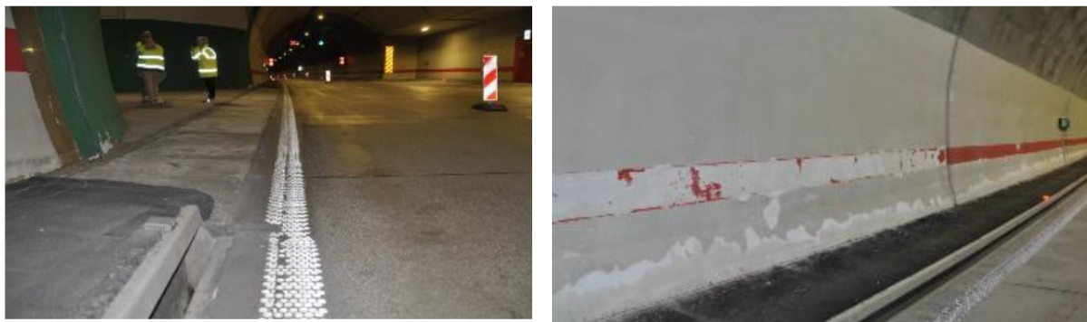
Figure 4. inadequate visibility and damaged or faded signage
