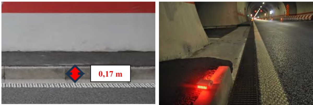
Figure 2. High curbs and unsafe edge of the evacuation path
