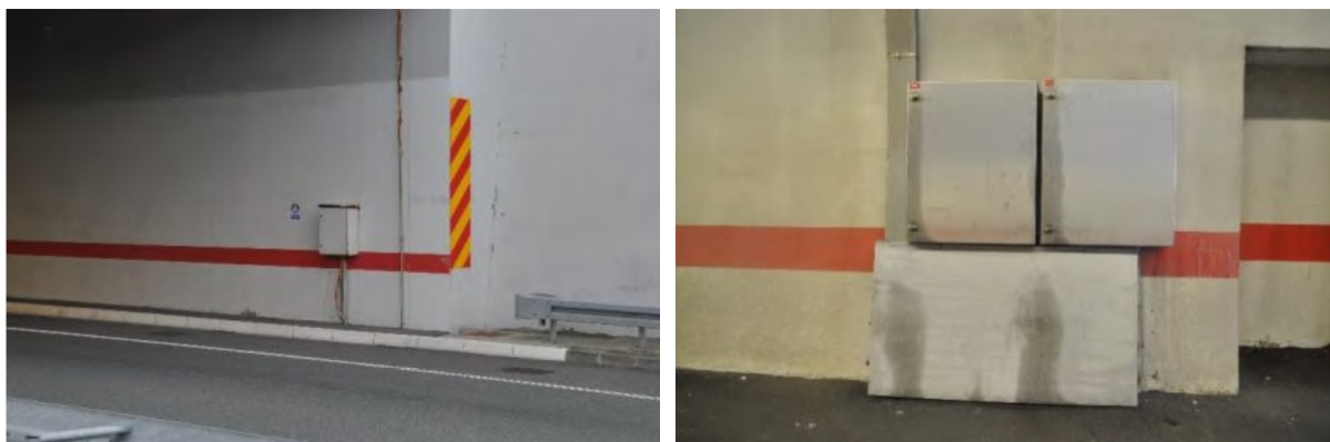
Figure 3. Unsafe positioning of electrical and control cabinets in the traffic zone
